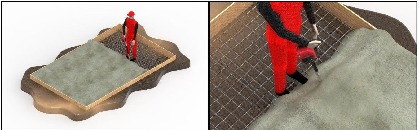
Figure 6: Operation procedure during the compacting of concrete.
