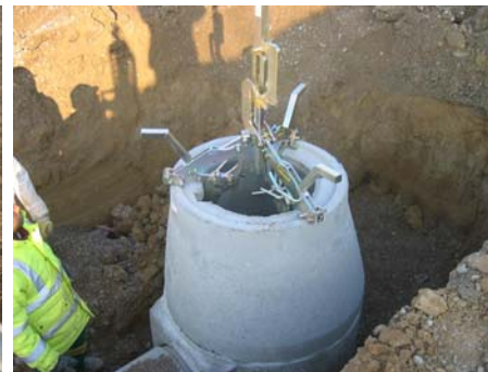
Also cone handling is not a problem for the installation clamp SVZ-uni .
