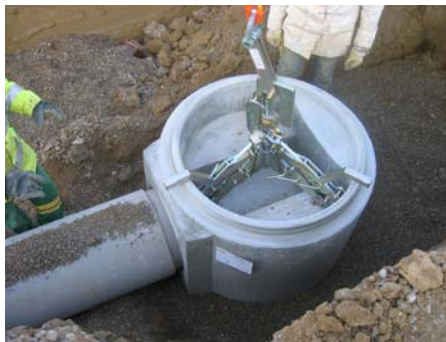
Economic installation of manhole basers
